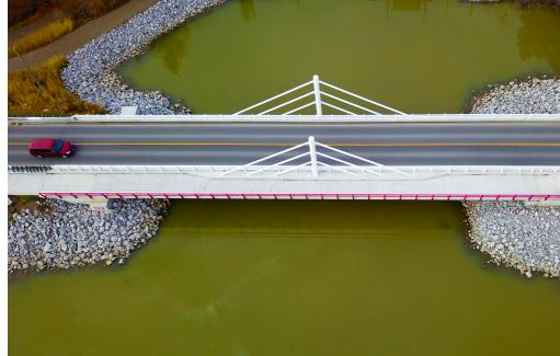
The bridge's superstructure comprises two very slender 500 mm-deep steel box girders, a series of transverse steel floor beams, and a composite cast-in-place concrete deck. The box girders are supported by steel pipe stays and pylons, the provision of which enabled the slender box girder design, allowing the structure to meet flood requirements without a significant grade raise to the existing road.
