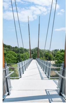
The Milne Dam Pedestrian Bridge is a multi-span, cable-stayed structure spanning the environmentally sensitive Rouge River in Markham, Ontario. The 45-metre main span crosses above the Milne Dam and features a fanned cable design with architecturally tapered steel pylons founded over 20 metres below the cable anchor points.
